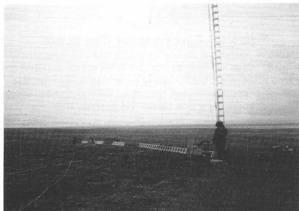
Figure 5: Erecting a 100 Foot Syledis navigation tower.
