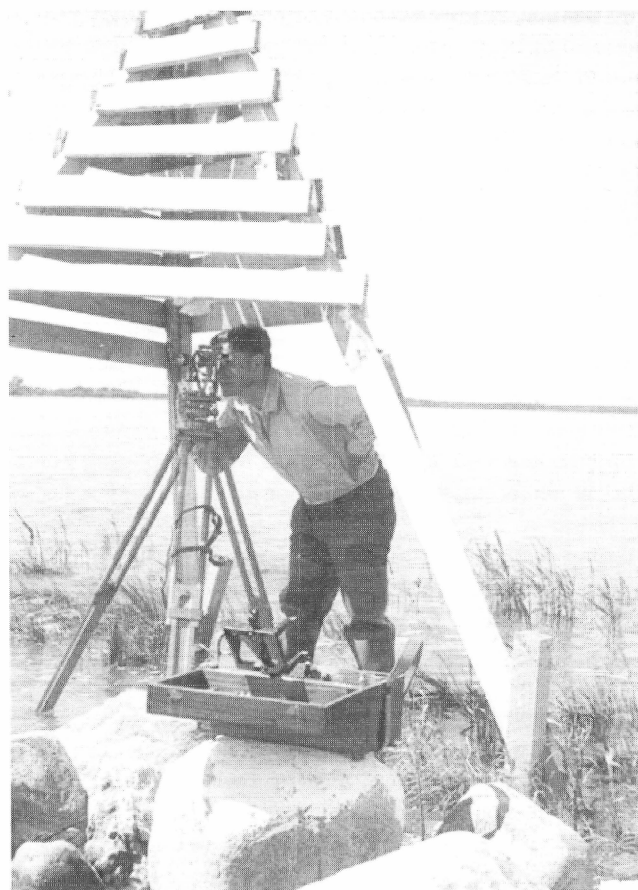
Sid van Dyck observing angles at a main triangulation station.
